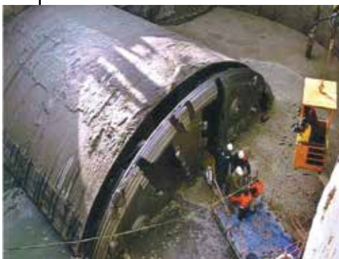
Left: TBM arrival in an inundated reception shaft
